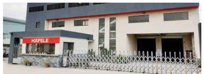
Häfele Production Plant Binh Duong, Vietnam
